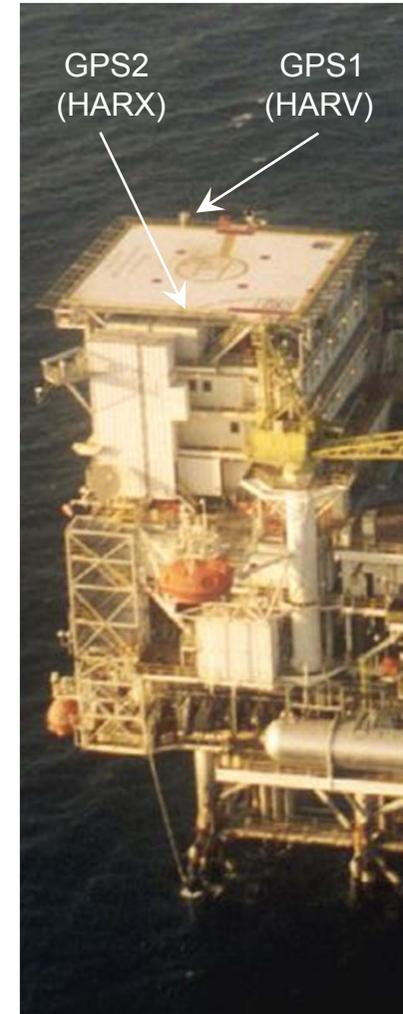
\*Independent GPS system (receiver + antenna) installed in 2015 for monitoring purposes.
