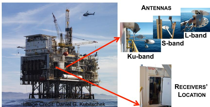
**Figure 1:** This figure shows the location of antennas and receivers at Platform Harvest. The antennas are located at approximately 27 meters above the ocean surface.
