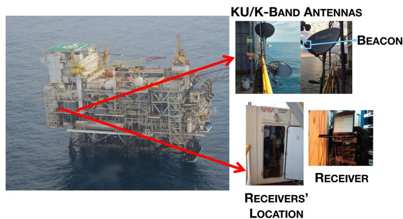
**Figure 1:** This figure shows the location of antennas and receivers at Platform Harvest. The antennas are located at approximately 27 meters above the ocean surface.
