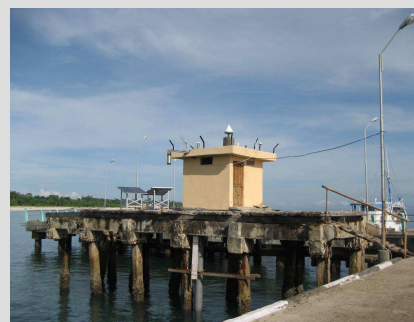
Example of a CGPS@TG station at Weikelo/Indonesia
